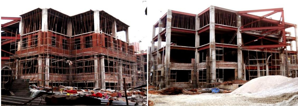
In a composite column both the steel and concrete would resist the external loading by interacting together by bond and friction. Supplementary reinforcement in the concrete encasement prevents excessive spalling of concrete both under normal load and fire conditions.
