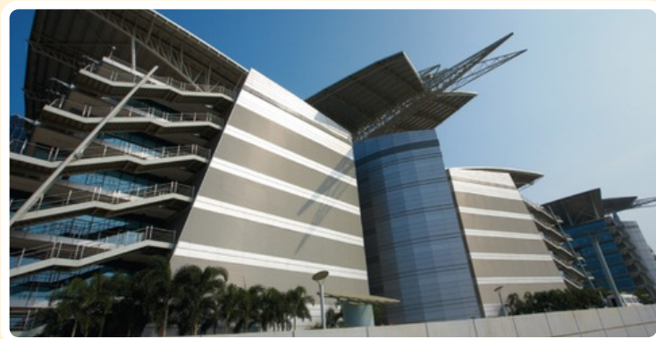
Fig 44 : TCS Technopark Building Chennai
