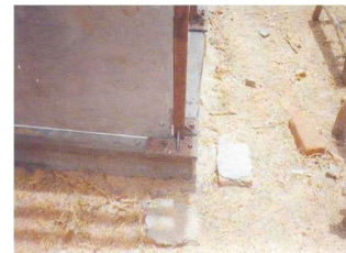
Connection of SHS with Ferro cement panel
