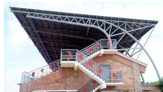
Galvanized pipe Steel cantilever Truss – Roof Structure
