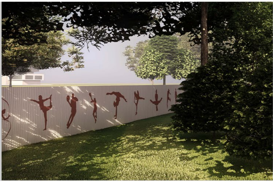
The Exterior boundry walls are being installed with different sport action motifs made of steel Plates.
