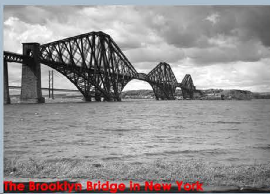
The Brooklyn Bridge in New York
