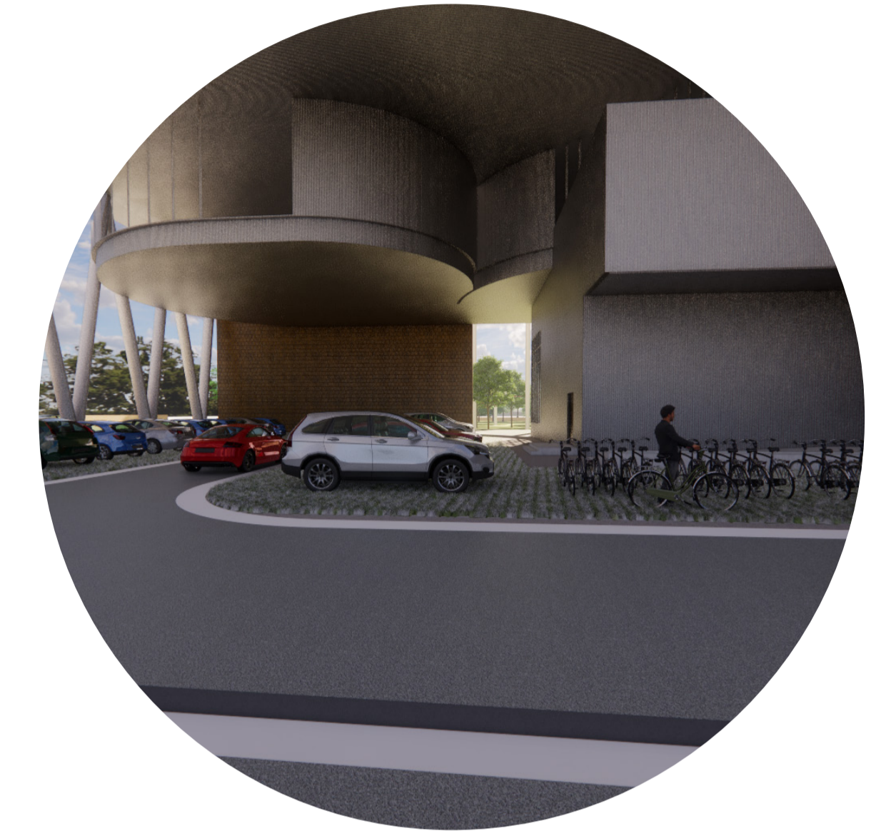
HANGING CONFERENCE HALLS FROM THE TRUSS BEAM OF AUDITORIUM SUPPORTED ON STRUTS
